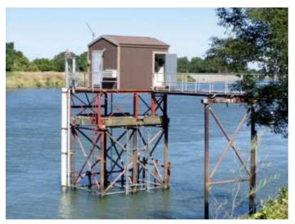
Figure 5. Sampling station on the Sacramento River at Hood, a key real-time monitoring station located within the Freshwater Boundary Region. Grab sample data at Hood and Greene's Landing (also on the Sacramento River) were used to characterize the Freshwater Boundary Region.
